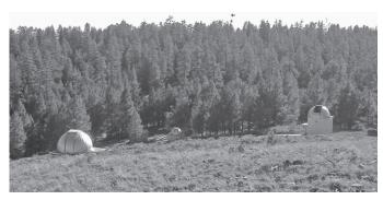
Figure 1: Pine Mountain Observatory's telescope facilities. The dome on the left houses a 32-inch telescope, the middle dome contains a 15-inch telescope, and the right dome has a 24-inch Boller and Chivens telescope.
