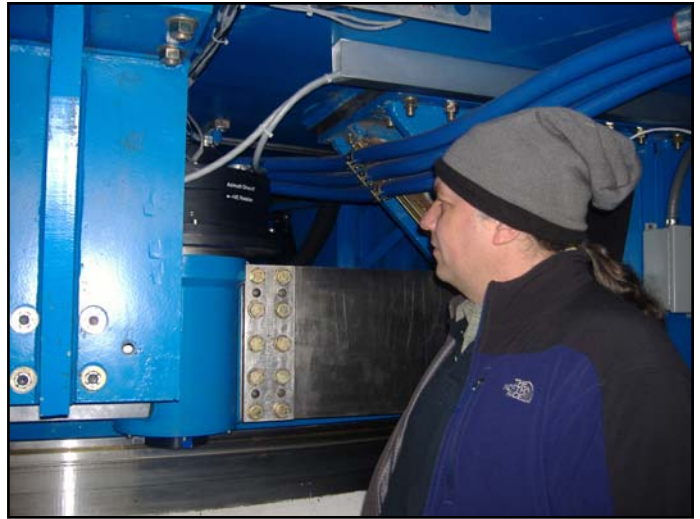
Dan examines the flex plate and azimuth high torque motor. Dan's cap helped keep him warm. The interior is kept at the expected nighttime temperature.
